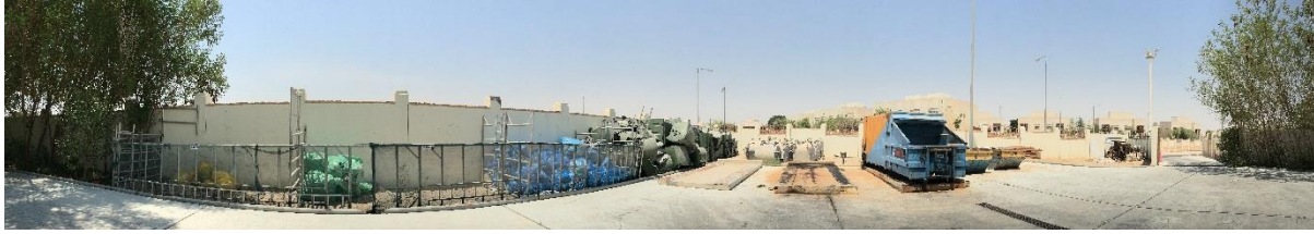
Figure 17: Lot 2 Waste Yard
