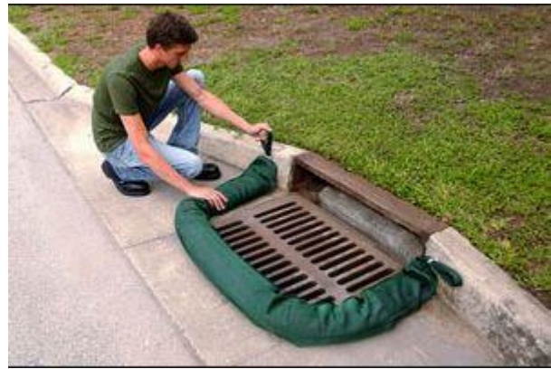
Figure 16 – Wattles Around Storm Drain
